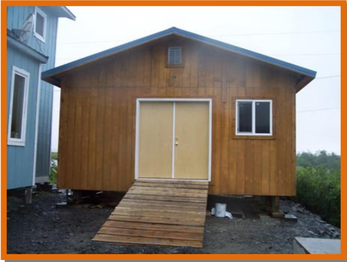
Final photo of completed construction
